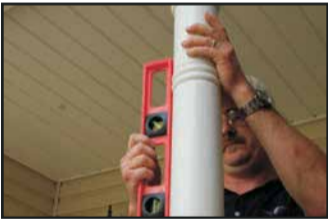
Step 9: Check post with level and remove temporary support.
