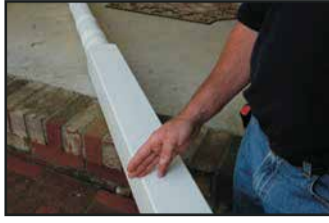
Step 2: Determine how much is to be trimmed (deduct 3/8 in. total to accommodate top and bottom mounting plates).
