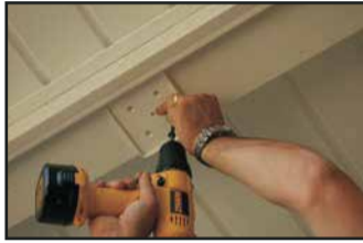
Step 4: Install ceiling plate.
