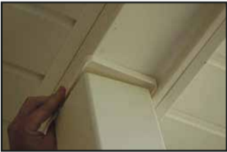
Step 7: Position top of post with top plate.
