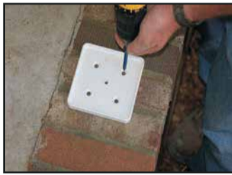
Step 6: Install bottom plate.
