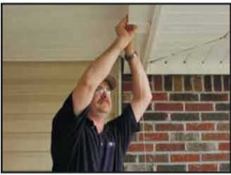
Step 5: Using a plumb tool, find and mark bottom position on floor.
