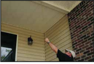
Step 1: Measure Opening to determine post length.
