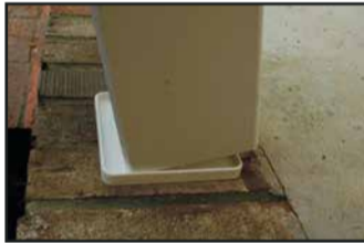
Step 8: Set post on bottom plate.
