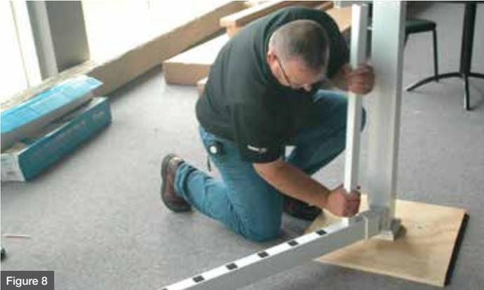
10. Remove the top rail and install the pivot brackets on the post following the same procedure as the bottom pivot bracket (Fig. 12 & 13).
