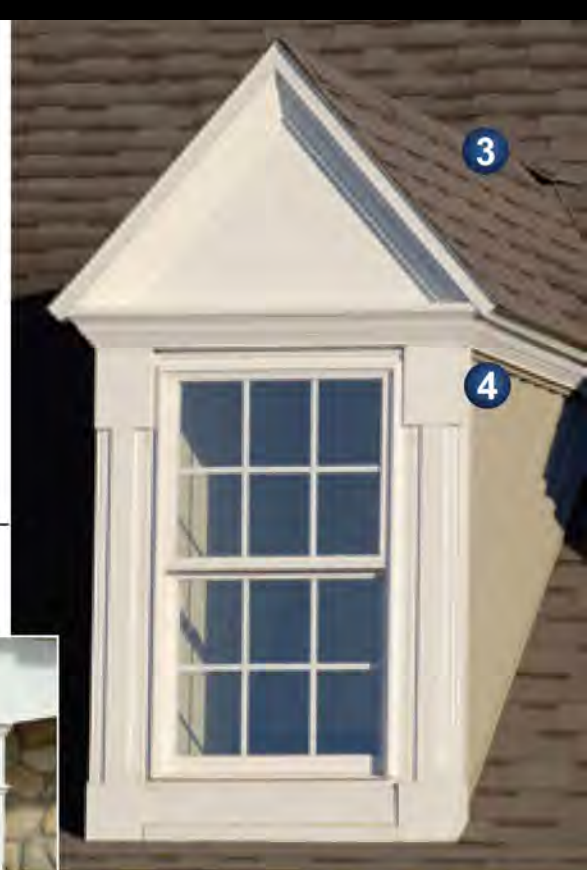
(Above) Dormer windows receive special attention on this house with urethane pediments, side trim and returns. (Left) Front porch header wrap fabricated from cellular PVC adds a customized look to the exterior of the home. (Below) Low-maintenance Fypon urethane and cellular PVC products add curb appeal and selling power to this Ohio home.
