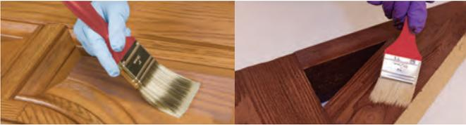
Stir the topcoat well with a stir stick. **DO NOT SHAKE.** Shaking causes bubbles in the topcoat and can cause improper application. The topcoat is milky in appearance but will dry clear.
