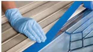
It is recommended that you clean the glass of any debris before staining. Mask off any glass and hardware.
